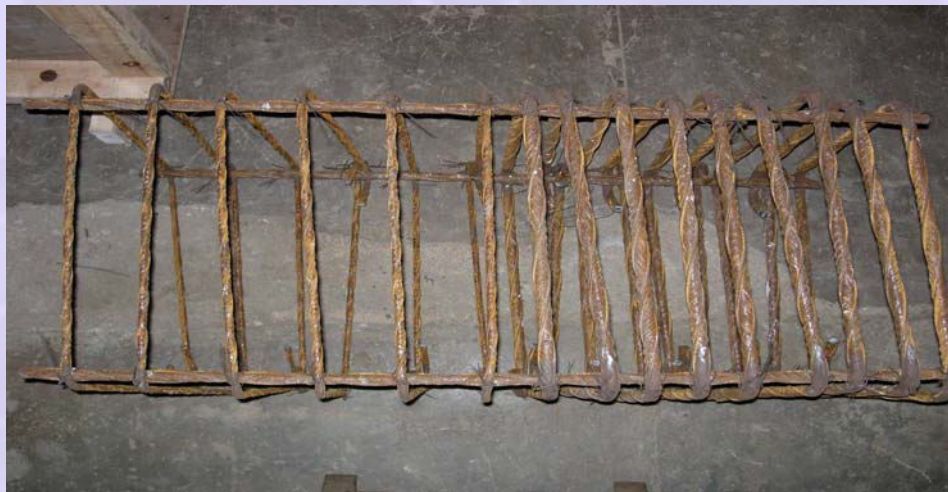
(a) Fabrication of end zone reinforcement
