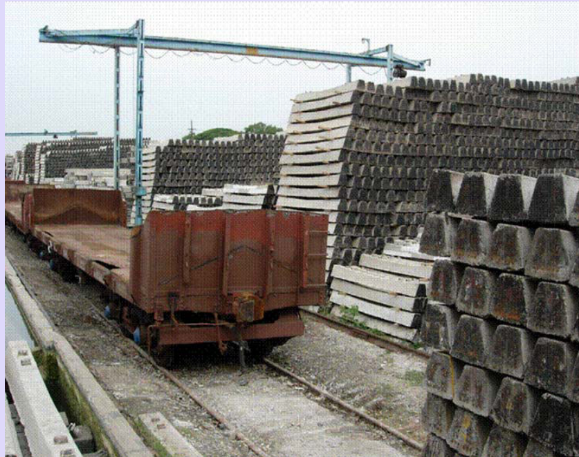
(n) Storage and dispatching of sleepers
