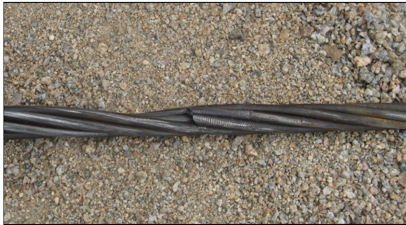
Photo 9.5: Broken prestressing wires due to prestressing wedges being too hard and damaging the strand
