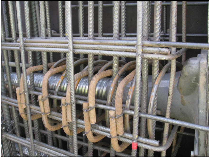
Photo 9.1: Reinforcement at prestressing anchor. The spiral behind the anchor is detailed by the prestressing supplier while the clips are detailed by the designer. Note that the clips should be anchored around a bar of its own diameter.
