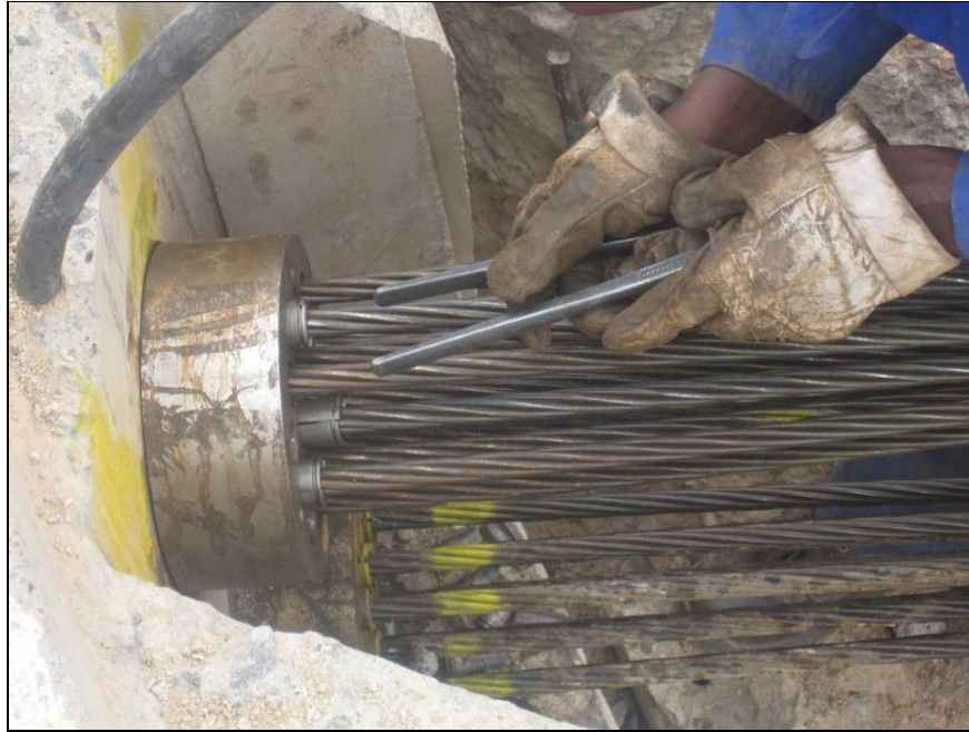
Photo 9.3: Seating prestressing wedges: This is best done with a tube around the strands rather than as seen in the photograph
