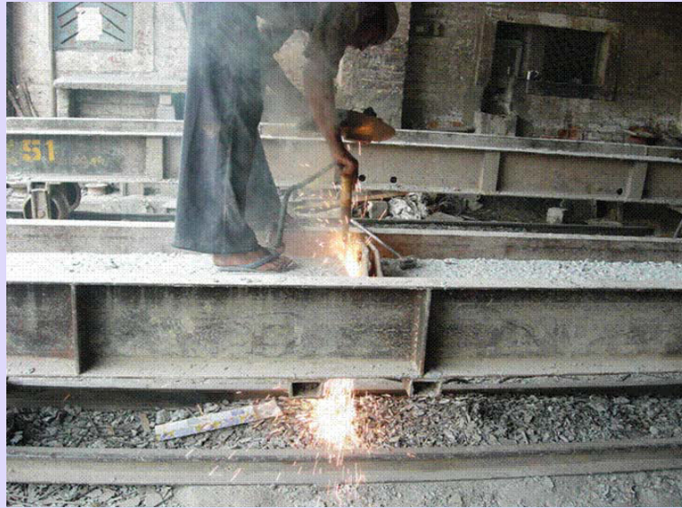
(j) Cutting of strands
