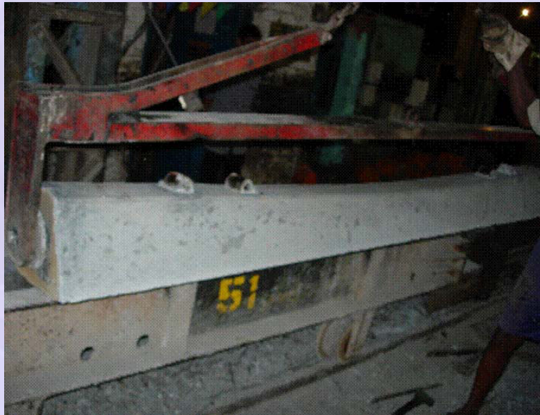
(k) Demoulding of sleeper
