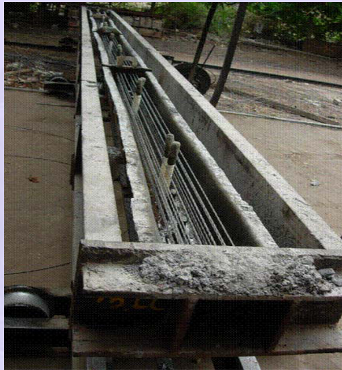
(a) Travelling pre-tensioning stress bench
