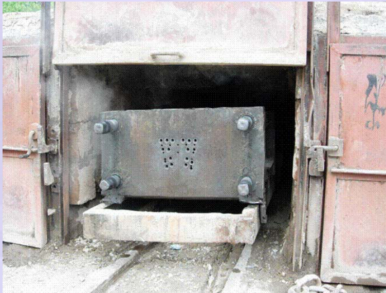
(i) Steam curing chamber
