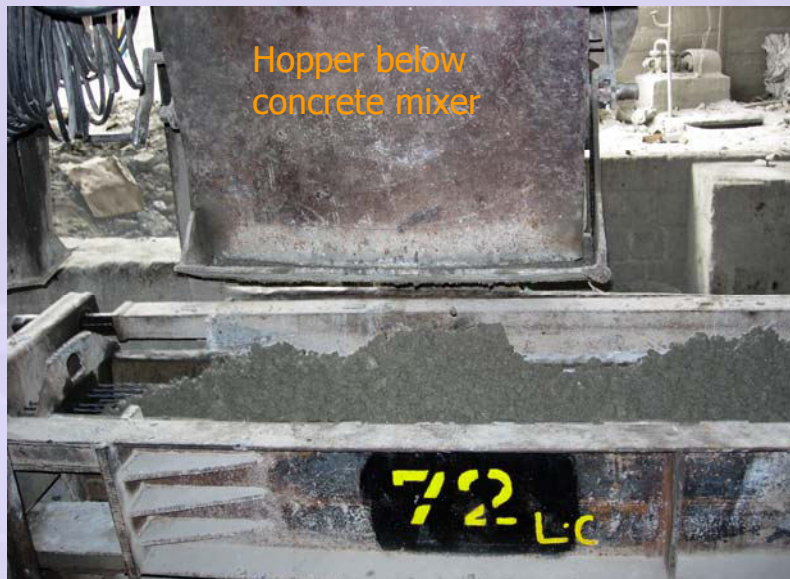
(g) Pouring of concrete
