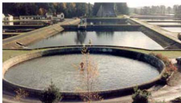
Figure 2-19: Sewage oxidation ponds
