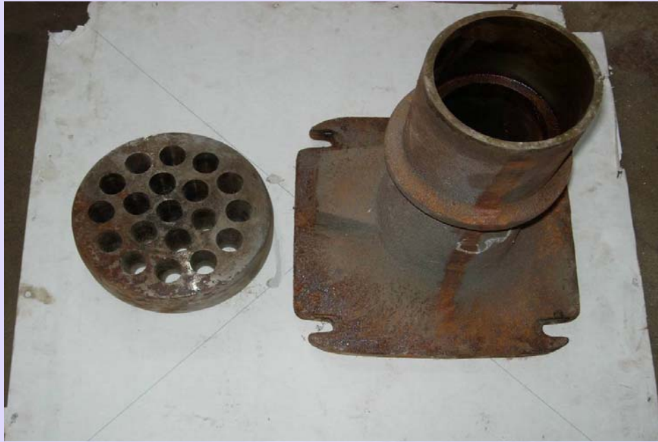
(b) Anchorage block and guide
