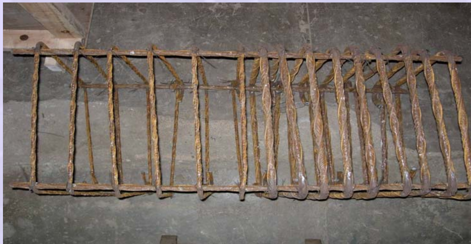
(a) Fabrication of end zone reinforcement
