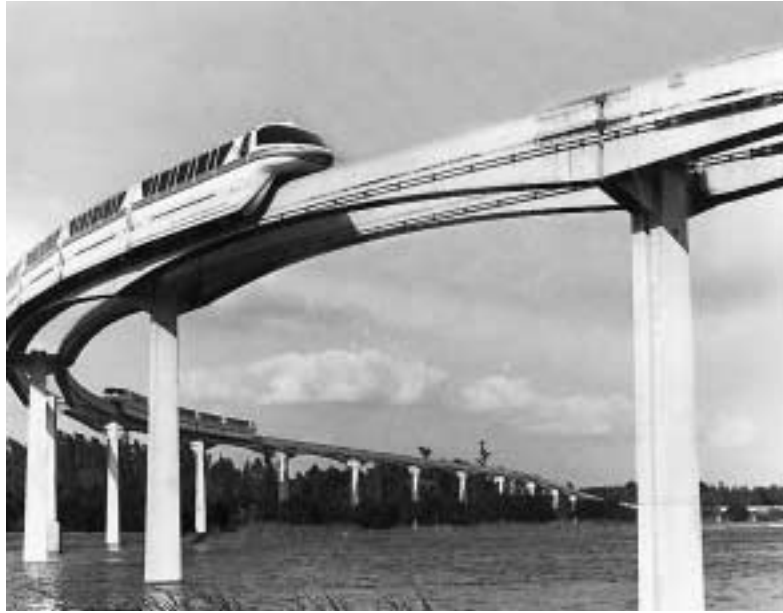
Photo 1.11 Walt Disney World Monorail, Orlando, Florida. A series of hollow precast prestressed concrete 100-foot box girders individually post-tensioned to provide six-span continuous structure. Designed by ABAM Engineers, Tacoma, Washington. (Courtesy, Walt Disney World Corporation.)
