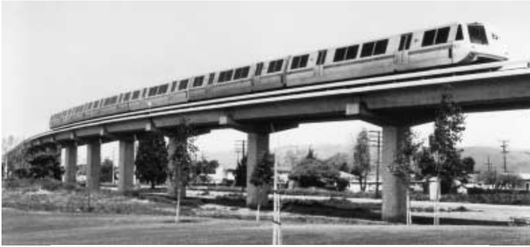
Photo 1.1 Bay Area Rapid Transit (BART), San Francisco and Oakland, California. Guideways consist of prestressed precast simple-span box girders 70 ft long and 11 ft wide. (Courtesy, Bay Area Rapid Transit District, Oakland, California.)
