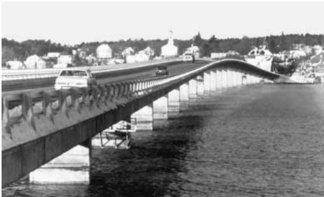
Photo 1.4 Wiscasset Bridge, Maine. (Courtesy, Post-Tensioning Institute.)
