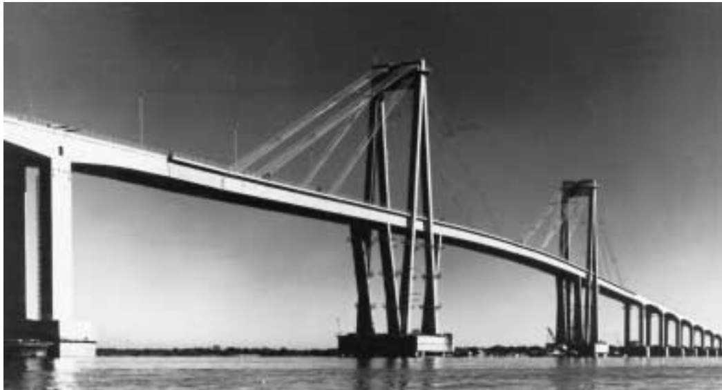
Photo 1.2 Chaco-Corrientes Bridge, Argentina. The longest precast prestressed concrete cable-stayed box girder bridge in South America. (Courtesy, Ammann & Whitney.)
