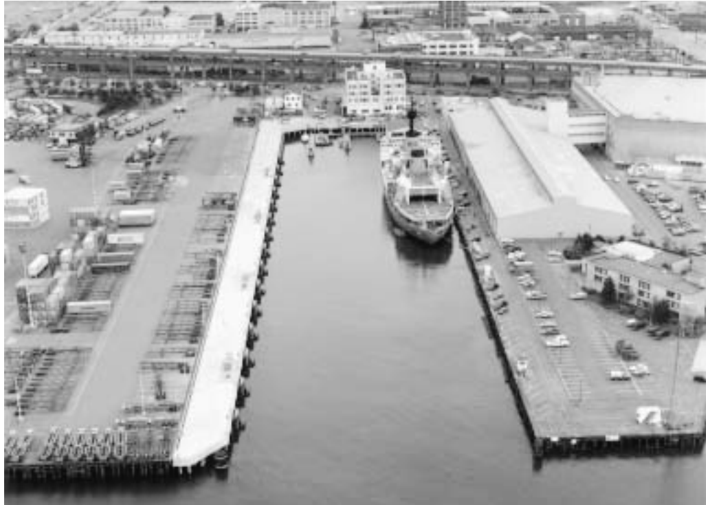
Photo 1.16 Pier 37 Rebuild, Seattle Washington: a 1200-ft-long by 40-ft wide pier consisting of 20-ft-long prestressed concrete deck panel supported by situ-cast concrete pile caps and prestressed concrete piles (Designed by BERGER/ABAM Engineers, Federal Way, Washington, courtesy Robert Mast, Chairman)
