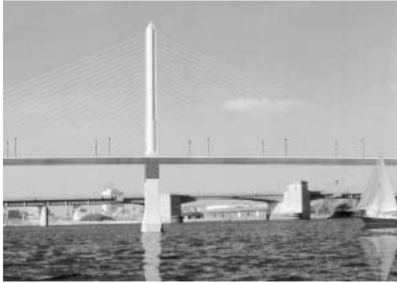
Photo 1.18 Rendering of the New Maumee River Bridge, Toledo. The design includes a unique single pylon clad with glass emitting LED arrays at night, single plane of stays, and a main span of 612 feet in both directions. Courtesy of the designer, FIGG Engineers of Tallahassee, Florida.
