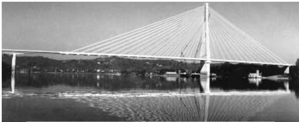
Photo 1.10 East Huntington Bridge over Ohio River. A segmentally assembled precast prestressed concrete cable-stayed bridge spanning 200-900-608 ft. (Courtesy, Arvid Grant and Associates, Inc.)
