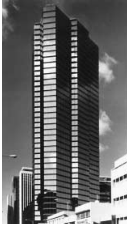
Photo 1.5 Executive Center, Honolulu, Hawaii. ( Courtesy, Post-Tensioning Institute. )
