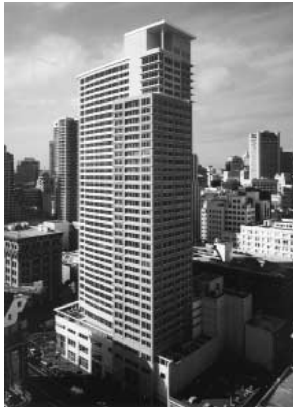
Photo 1.17 Paramount Apartments, San Francisco, CA: the first hybrid precast prestressed concrete moment-resistant 39 floor high-rise frame building in high seismicity zone, 2002. (Courtesy Charles Pankow Ltd., Design/Build contractors. Structural Engineers: Robert Englekirk Inc.; Design Architects: Elkus/Manfredi; Executive Architect: Kwan Henmi, Inc.; Owner: The Related Companies)
