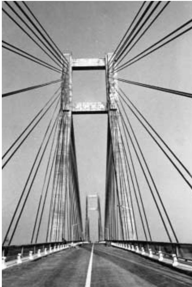
Photo 1.9 Tianjin Yong-He cable-stayed prestressed concrete bridge, Tianjin, China, the largest span bridge in Asia, with a total length of 1,673 ft and a suspended length of 1,535 ft, was completed in 1988. (Credits Owner: Tianjin Municipal Engineering Bureau. General contractor: Major Bridge Engineering Bureau of Ministry of Railways of China. Engineer for project design and construction control guidance: Tianjin Municipal Engineering Survey and Design Institute, Chief Bridge Engineer, Bang-yan Yu.)
