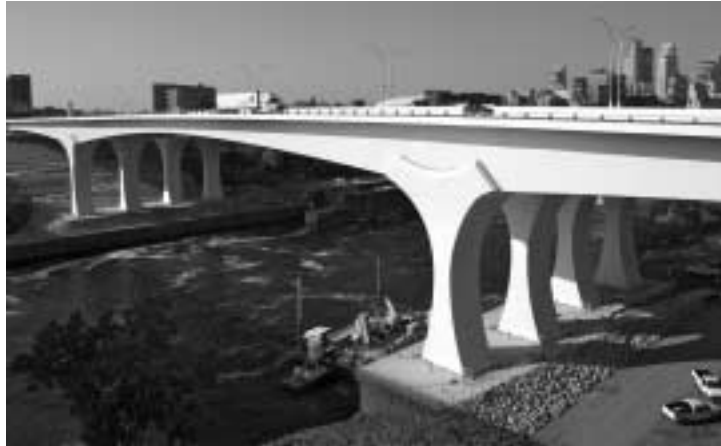
Photo 1.8 The new I-35W bridge, Minneapolis, Minnesota. Designed by FIGG, the 10-lane interstate bridge has a 504' precast, prestressed concrete span over the Mississippi River, with 75' vertical clearance. The span's 120 precast concrete segments, each 45' wide, up to 25' deep and weighing 200 tons, achieved an average concrete strength of 7600 psi. These segments for the main span were assembled in one directional cantilever from the main piers in just 47 days. The bridge has 50,000 cubic yards of concrete and nearly 3 million pounds of post-tensioning steel that runs the length of the twin 1,214' bridges. This new interstate bridge was designed and built in 11 months, opening on September 18, 2008. (Courtesy of FIGG, the bridge designer)
