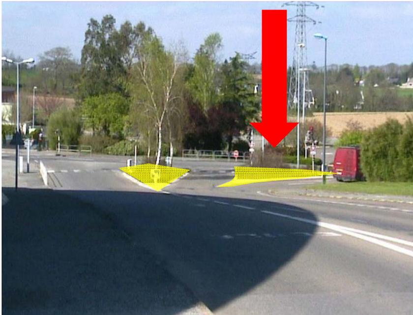
This method also has the advantage that it prevents overtaking in closer area of the intersection.
