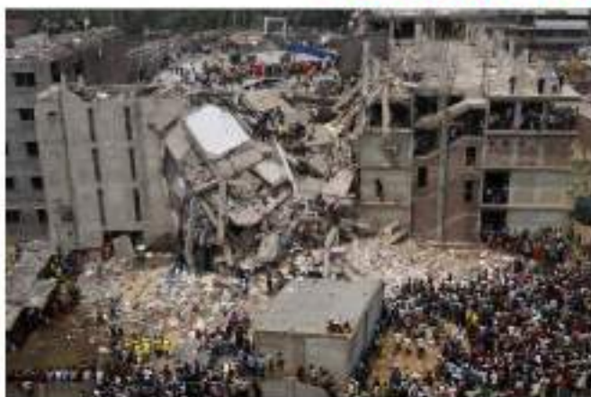
(a) Inadequate Strength
